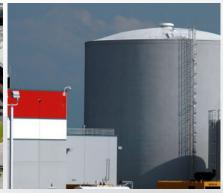
THERMAL ENERGY STORAGE TANKS WORK BY CAPTURING EXCESS HEAT OR COLD AND RELEASING IT WHEN NEEDED. HOT AND COLD TEMPERATURES ARE OFTEN CAPTURED THROUGH PERIODS OF HIGH PRODUCTION OR LOW DEMAND.
