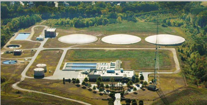
THREE (3) - 278'- 0" ID FREE-SPAN CONCRETE DOMES
