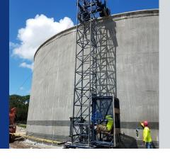
Both the core wall and the free-span dome roof are circumferentially prestressed using high-strength steel wire wrapped around the tank in a continuous helix. Wall prestressing is designed to carry the tank's hydraulic load, while dome ring prestressing resists the horizontal forces of roof live and dead loads.
