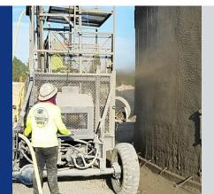
Exterior encasement of the steel shell is accomplished with shotcrete, which is pneumatically placed concrete. The core wall of the tank is constructed using successive layers of shotcrete until the required wall thickness is achieved.
