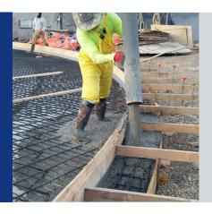
The floor of the prestressed tank is typically a heavily reinforced concrete membrane slab. Structural and ballast floor designs are also common depending on site condition requirements. This view illustrates placement of floor concrete, highly reinforced; a strong foundation.
