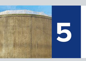
Vertical reinforcing bars are placed to design requirements and encased in shotcrete.
