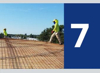
Once the dome formwork is completed with an overlay of sheathing, reinforcement is placed.
